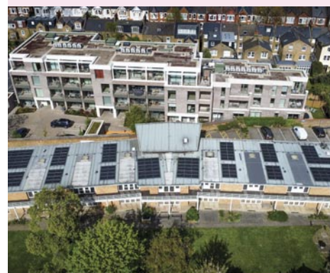
Solar panels on Minnie Kidd House
